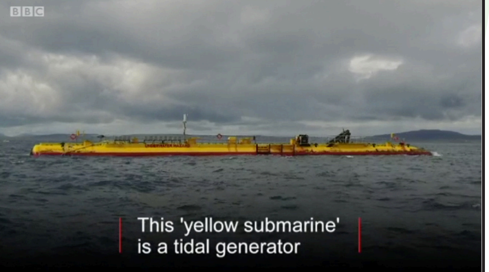
The SR2000 was installed in the Fall of Warness, west of the island of Eday, in August 2017
